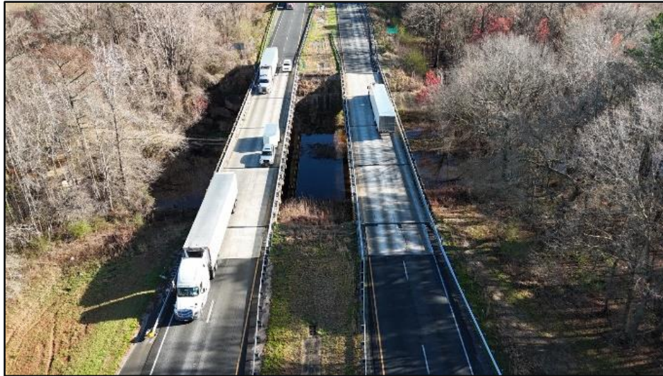
Bridge Nos 000000001010082 and 000000001010082 Over Black Creek
