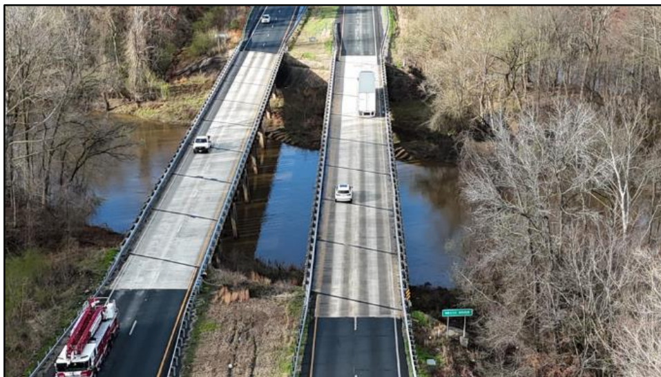
Bridge Nos. 000000001010100 and 000000001010101 Over Neuse River
